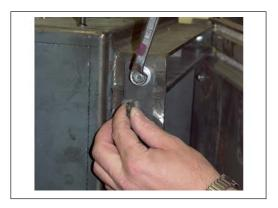
☐ Adjust the contact pressure on the door handle side on the locking plate
